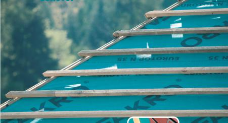
**EUROTOP** membranes are characterised by a unique combination of features such as water-tightness and water vapour permeability.
